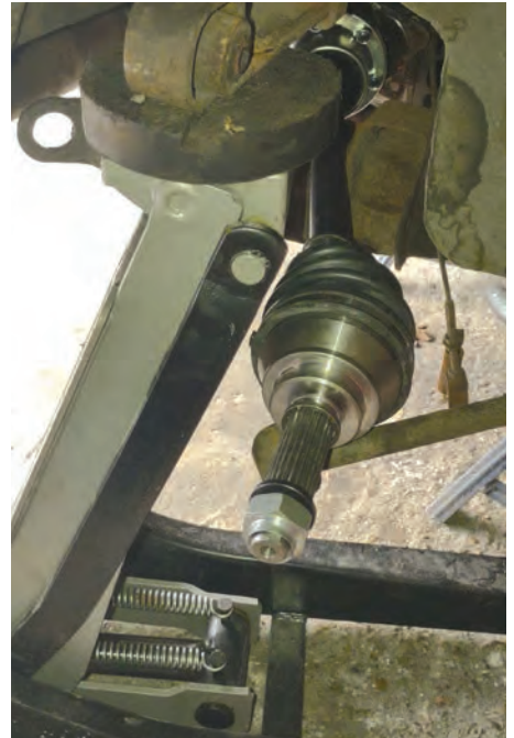
12. Getting the shaft into place using a jack on the spring to provide space.
